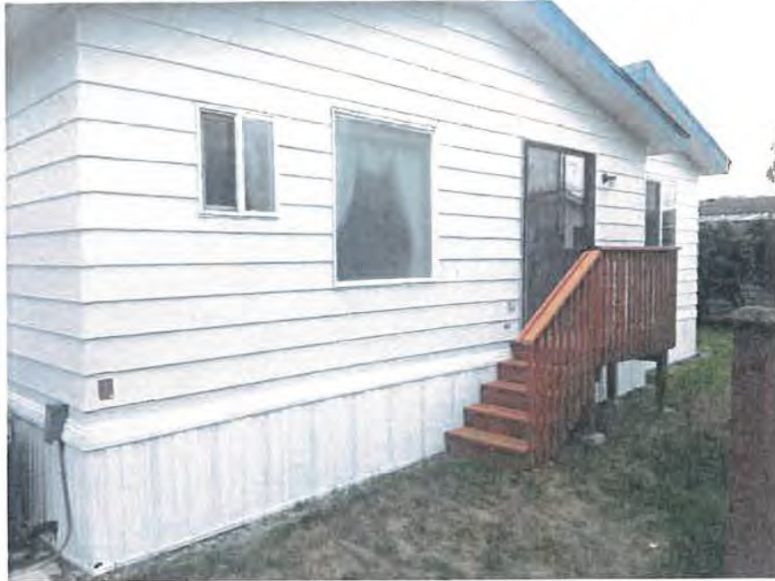
REAR VIEW - LOOKING AT WEST SIDE - Photo Taken 9-17-2013
