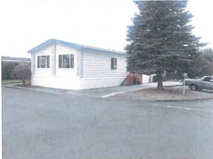
SIDE VIEW - LOOKING AT NORTH SIDE - Photo Taken 9-17-2013
